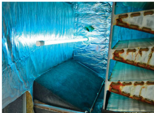
FEELING BLUE: Both residentially and commercially, UV light is being used to combat germs, bacteria, viruses, mold, and fungi.
